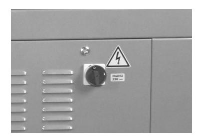
On/off switch is located on front of electrical control panel.
